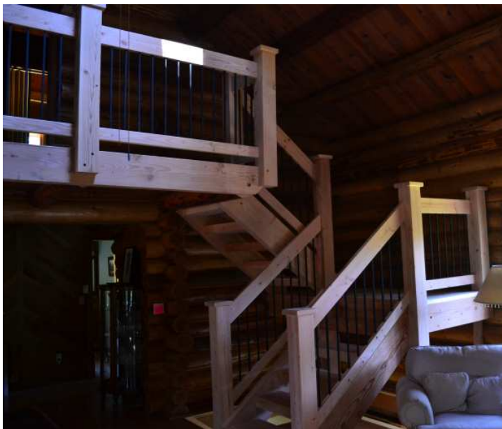
(below) Iron Rod Rail w/ Fir Dimensional Lumber
