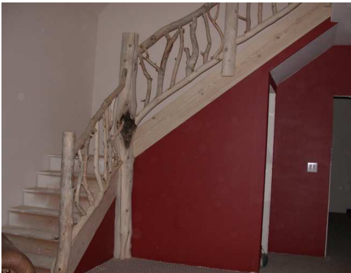
(below L&R) Branchwork Flat & Stair Rails
